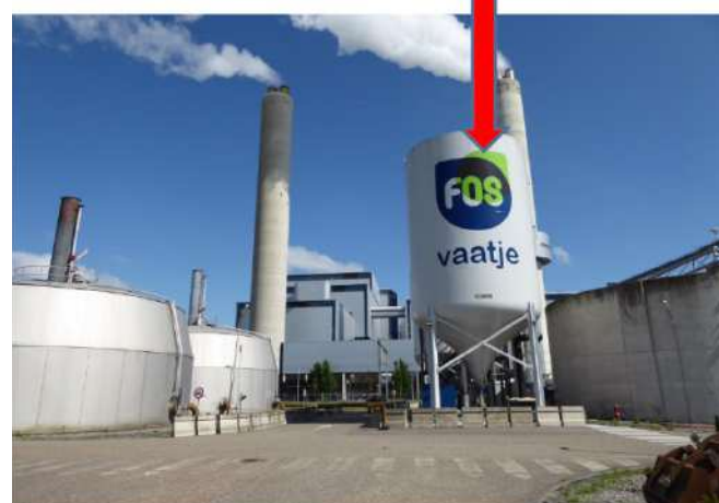
Figure 2: Magnesium recovery from a drinking water production reverse osmosis plant for struvite recovery from wastewater.
