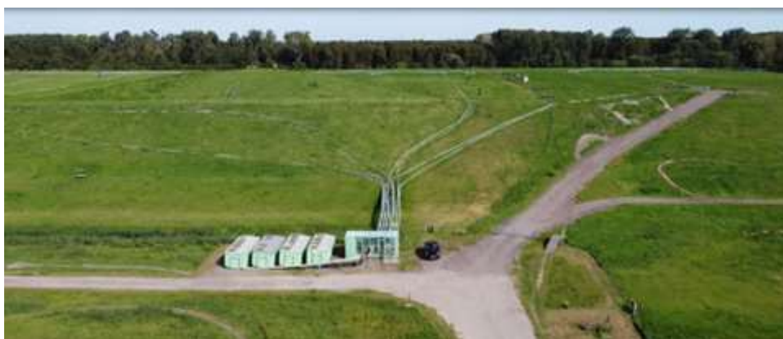
Figure 4: Landfill under aeration. Source: Afvalzorg.
